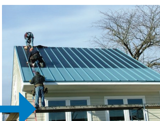
Work is in progress.
