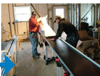
The roofing contractor completes the PV installation.
